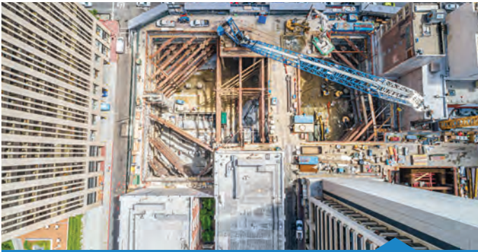
TEMPORARY WORKING TRESTLE AND LR1300 CRANE
