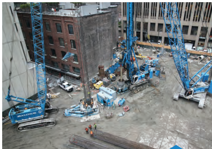
BG50 DRILLING OPERATIONS AND REBAR CAGE INSTALLATION
