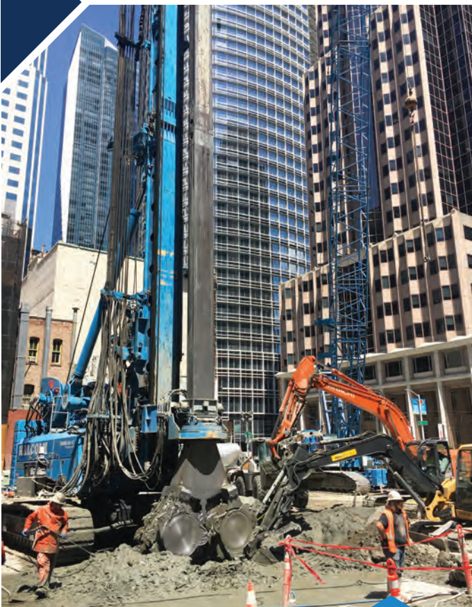
BG42 WITH CUTTER SOIL MIX ATTACHMENT
