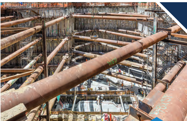
TOWER 1 INTERNAL TEMPORARY BRACING AND T1 NORTH ELEVATOR PIT
