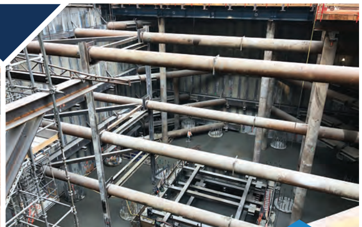
TOWER 2 INTERNAL TEMPORARY BRACING AND T2 ELEVATOR PIT
