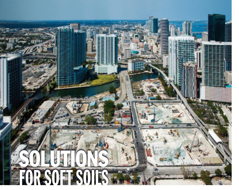
Because of poor soils, high water tables, and high wind and hurricane loads, deep foundations and basements in southeast Florida have been virtually impossible, limiting the heights of towers in cities like Miami. But thanks to contractor innovations—including cutter soil mixing, deep soil mixing, and continuous flight auger megapiles—robust underground support is now possible, and towers in and near Miami are rising.
