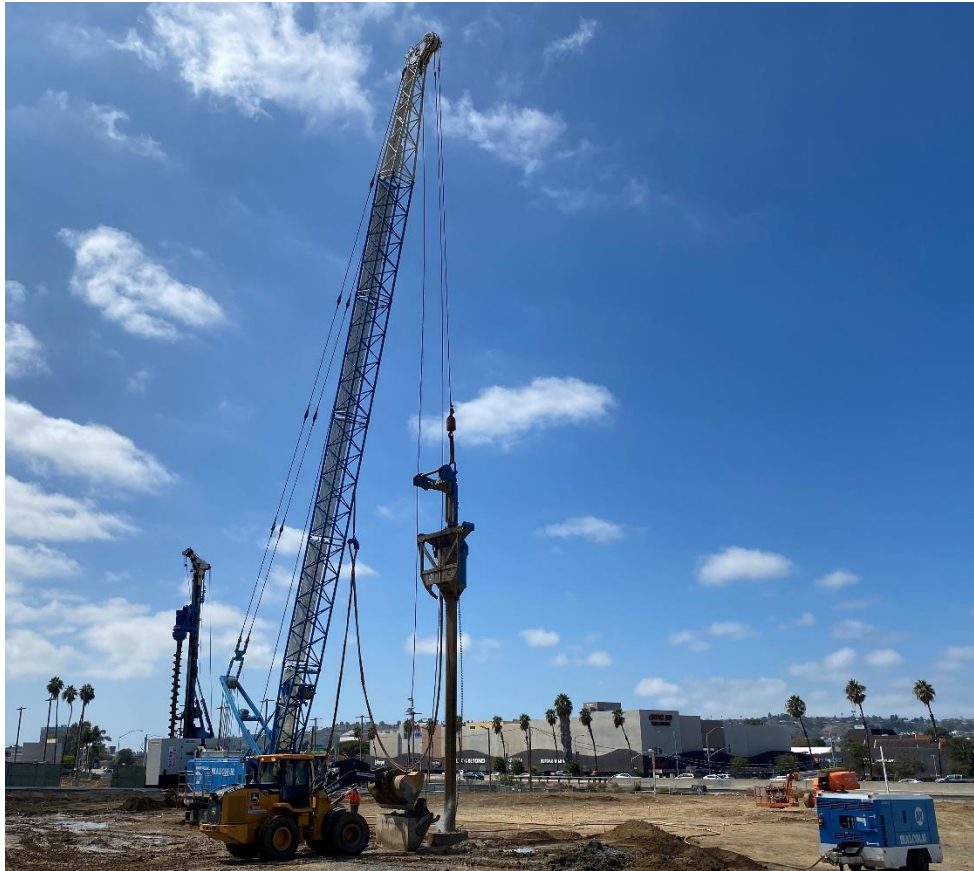
Fig. 5. Stone Column Installation at Site
