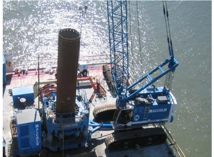
With over 1 million pounds of extraction force, the rotator was able to remove the temporary casing while maintaining as much as 40' of concrete above the bottom of the casing.
