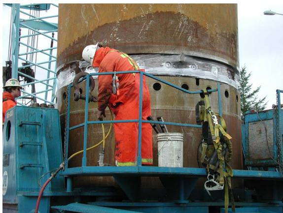
Figure 3. Joining the casing tubes.
