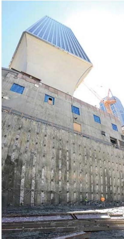
Matyasovszky led the tricky shoring-and-drilling operation that kept a deep pit from undermining a 40-story tower.
