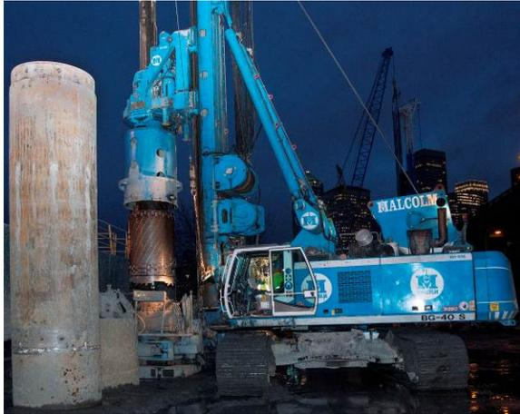
Figure 4: BG40 with 5 ft oscillator installing tangent pile wall
