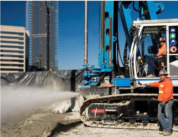
Figure 2: BG 15 with jet grouting attachment
