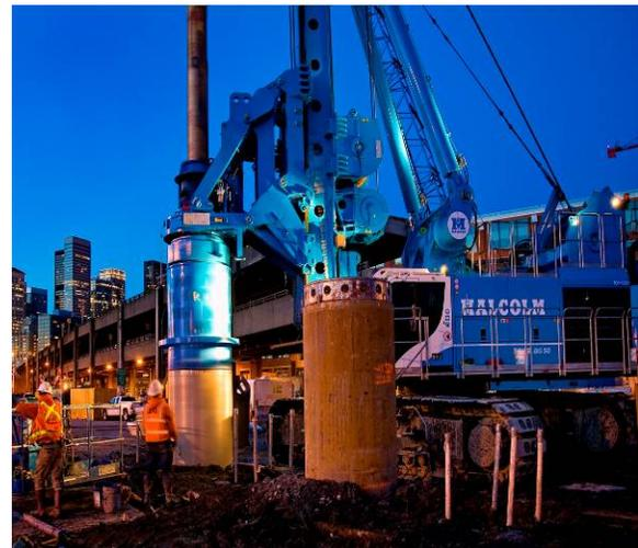
Figure 5: BG 50 installing 5 ft diameter secant pile wall
