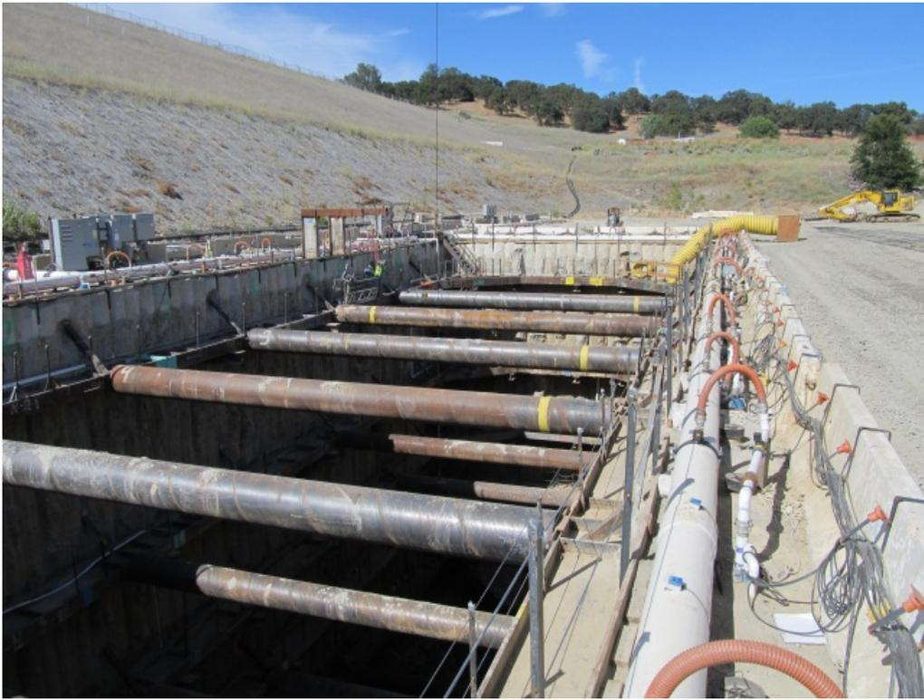
**Figure 5.** Photo of Internally-Braced Secant Pile Wall System Used for Key-Block Cell Construction with Dewatering Wells and Manifold System
