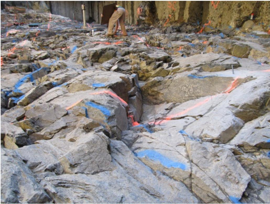
**Figure 6.** Photo of the Excavated and Cleaned Amphibolite Schist Bedrock Surface Being Mapped
