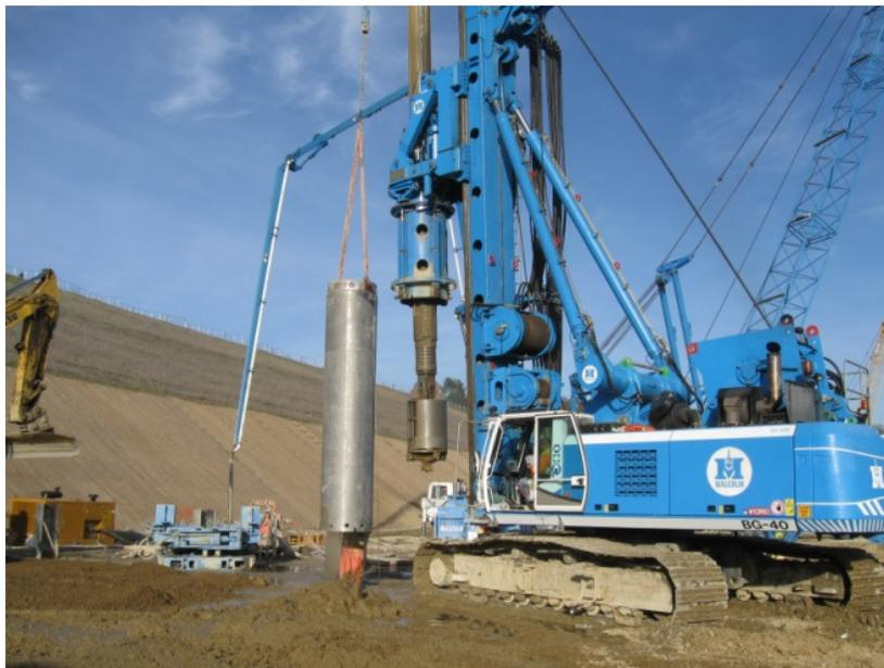
**Figure 3.** Top Drive Rotary Crawler Drill
