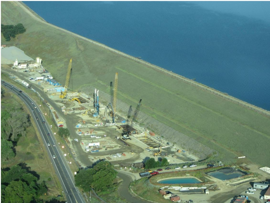
**Figure 7.** Aerial Photograph Showing Construction Underway at Two Key-Block Cells
