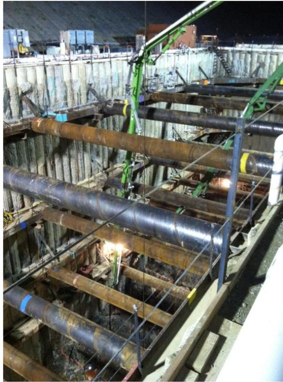
**Figure 8.** Key-Block Concrete Placement
