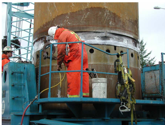
Figure 3. Joining the casing tubes.
