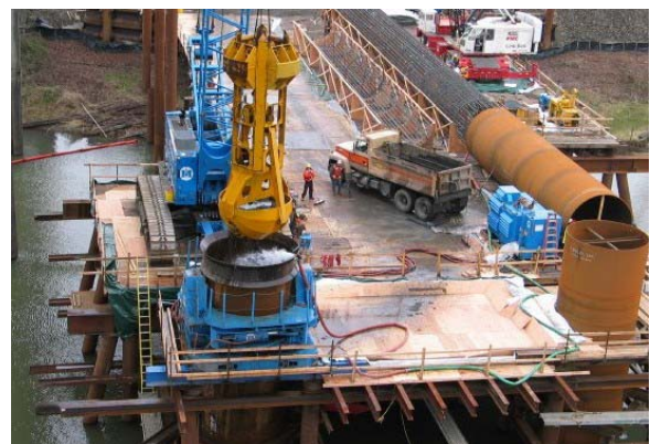
Figure 4. Excavation with spherical hammergrab and 3 meter casing oscillator.
