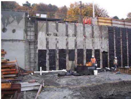
Figure 3. Completed CSM Wall
