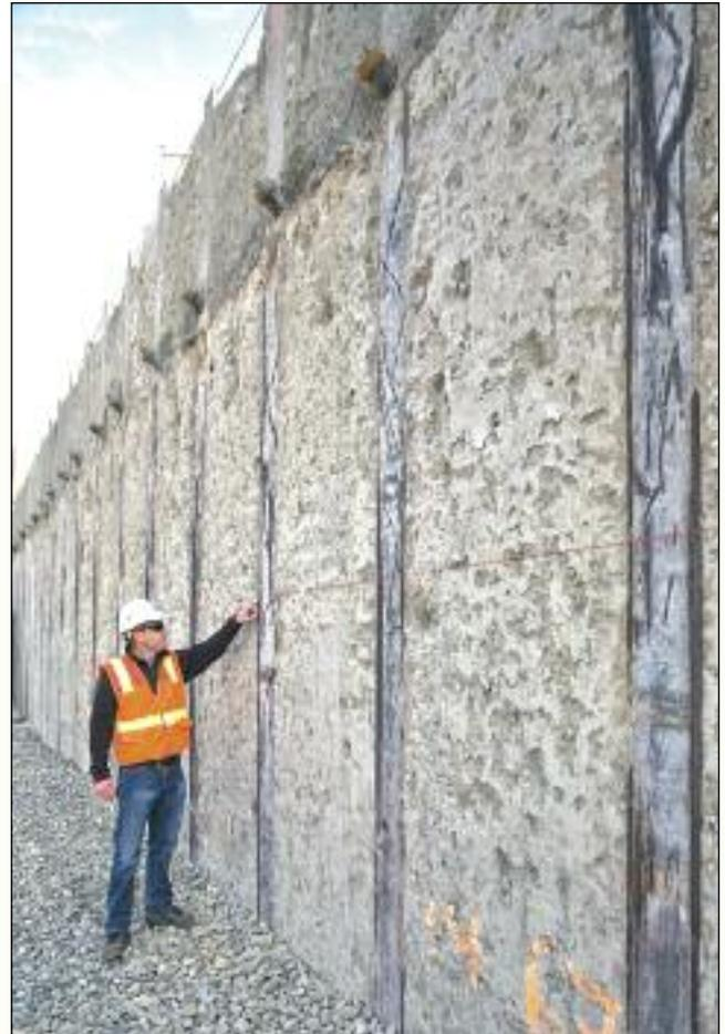
The engineer inspects the final product. Amazingly, very few leaks were encountered during excavation and in the event one was encountered MDCI crews would quickly repair them.
