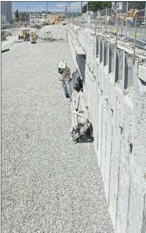
125,000 square foot site footprint excavated up to 14' below the water table, the success of MDCI CSM shoring allows for a dry site.
