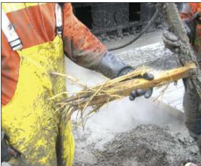
*The encountering of existing wood piles was a common occurrence on the Elliott site. The BCM 5 cutter head made quick work of these obstructions and the resulting shavings simply floated to the top and were removed with the spoils.*
