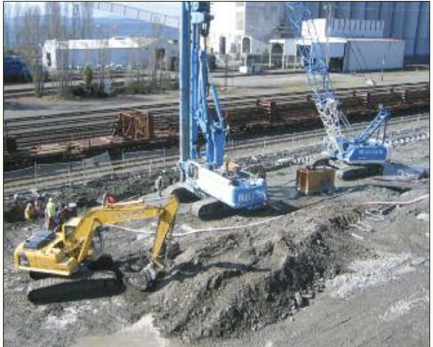
MDCI RTG 23 and Kobelco BM 500 Installing panels and piles along the Burlington Northern Railroad.
