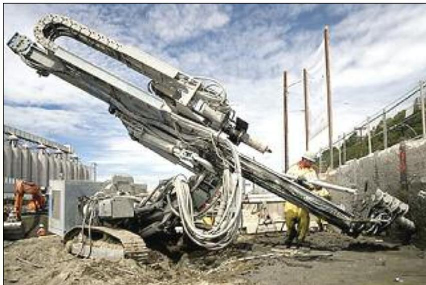
MDCI employee unloads drill steel while installing tiebacks through the Cutter Soil Mix Wall. After tieback installation, holes were plugged with chemical cement to stop the inflow of water.
