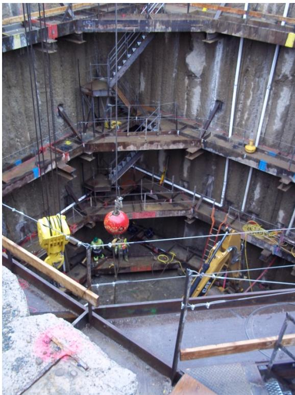
Figure 5: Key Block Excavation at 52 ft (16 m)
