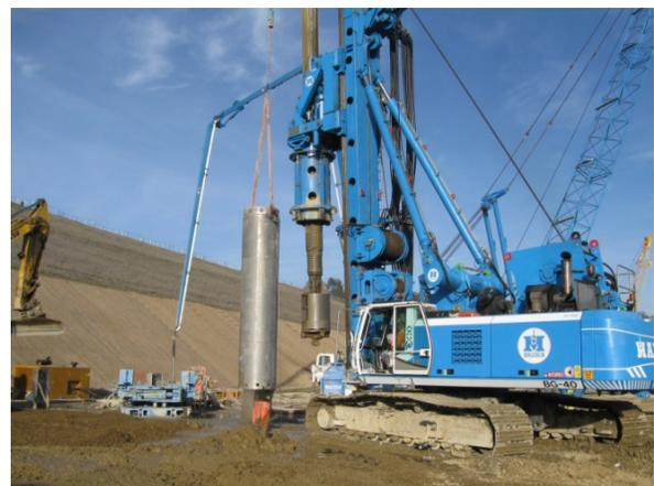
Figure 2: Drill Rig and Casing Oscillator
