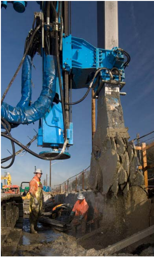
FIG. 6. CSM rig in operation.
