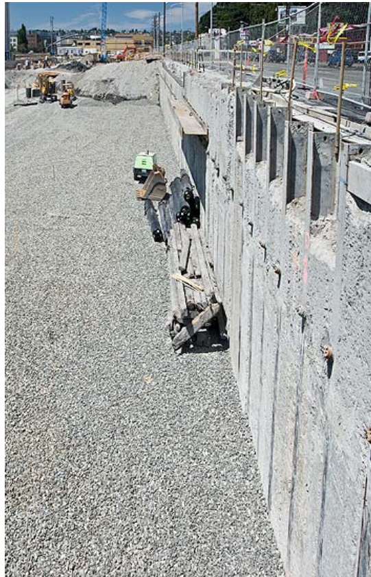
FIG. 7. Excavated soil mixed wall along Elliott Avenue.
