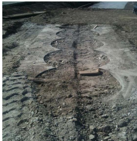
**FIGURE 5 – Completed Guide wall Section**
