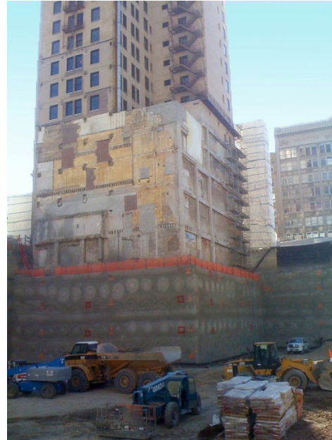
Figure 4: Photo of Shoring at Deseret Trust Building during Excavation
