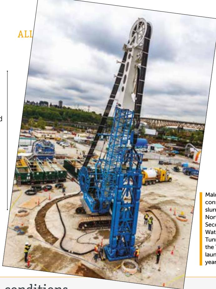
Malcolm-Petrifond constructed the slurry walls for the North shaft of the Second Narrows Water Supply Tunnel, from which the TBM is due to launch in May this year.
