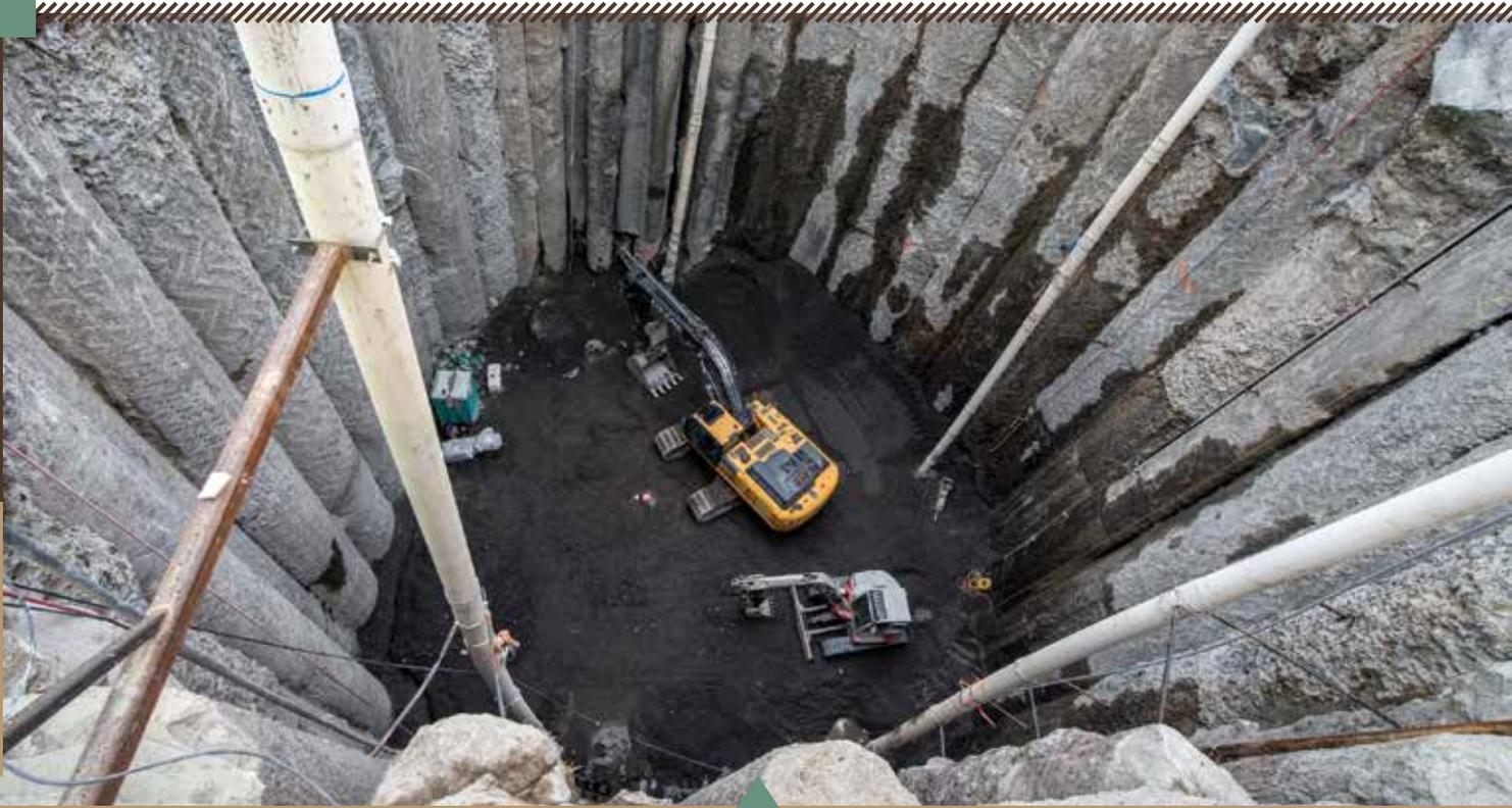
Access shaft for Bertha's rescue required dewatering wells on the interior and exterior of the shaft to control groundwater flow and pressure.
