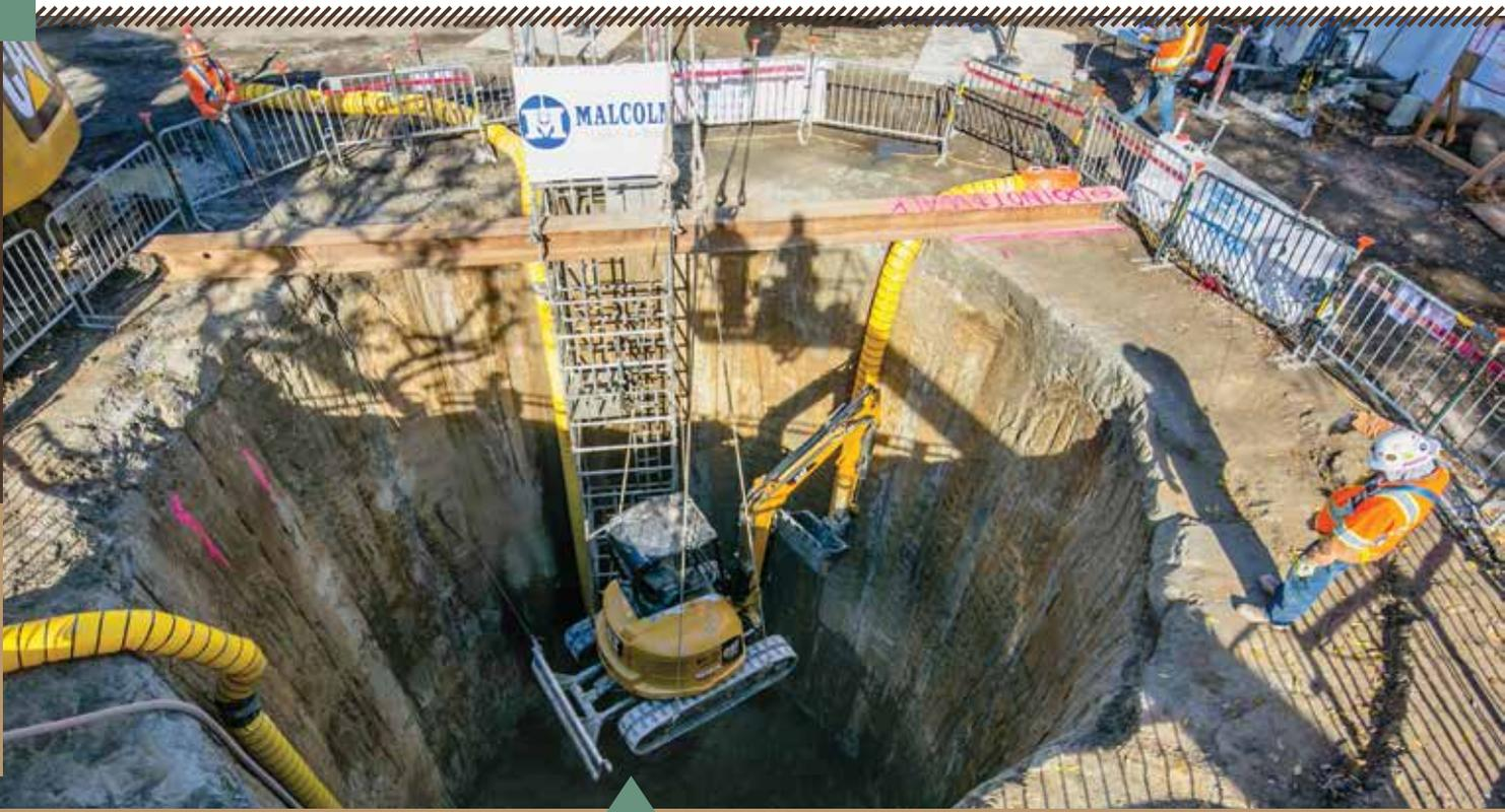
Cutter soil mixing walls were an economical and faster construction technique for micro-tunneling access shafts on PG&E's gas pipeline replacement project.
